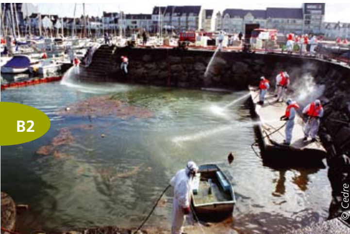
Cleaning riprap and the harbour basin as a result of pollution by heavy fuel oil. Port de la Turballe, France.
