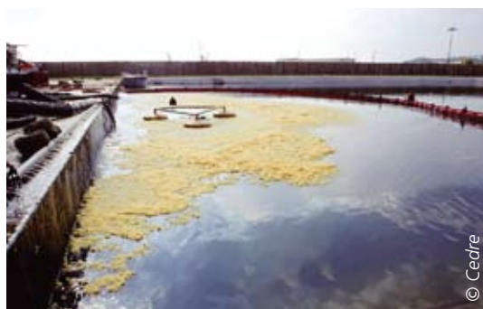
Using bulk sorbents to finish off mechanical recovery operations. Water curtain set up to protect a quay and recovery with a circular weir skimmer.
