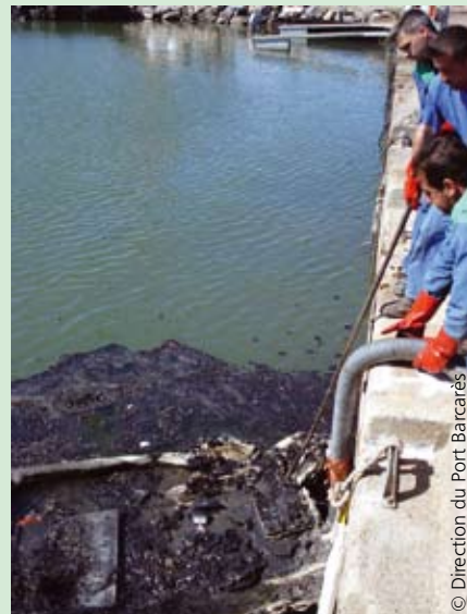
Pumping using vacuum trucks and manual recovery in a harbour basin.
