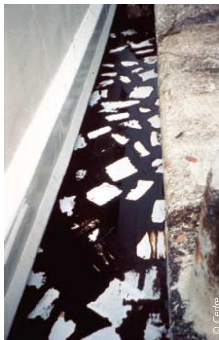
Sheet sorbent between a vessel and the quay.
